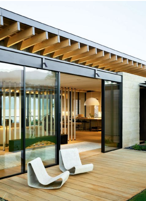
This page: Subtle sun control measures appear throughout the house. Series of louvered screens (some fixed and some pivoting) and clerestory windows topped by deep overhangs keep interiors protected from glare.
